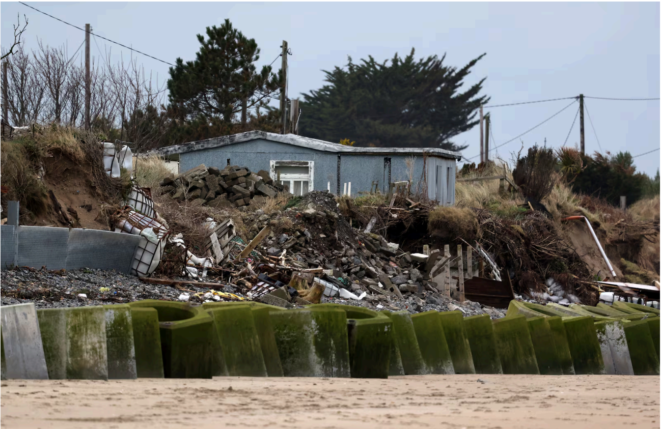
Eroded properties on Portrane beach, north Dublin. Photograph: Colin Keegan/Collins
